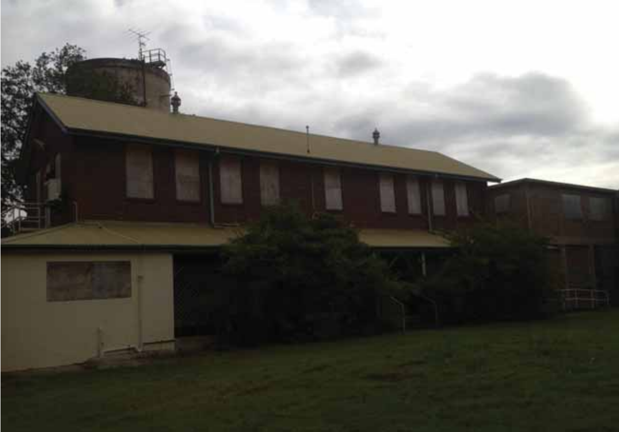
FIGURE 9 – SOUTHERN ELEVATION OF ADMINISTRATION BUILDING
