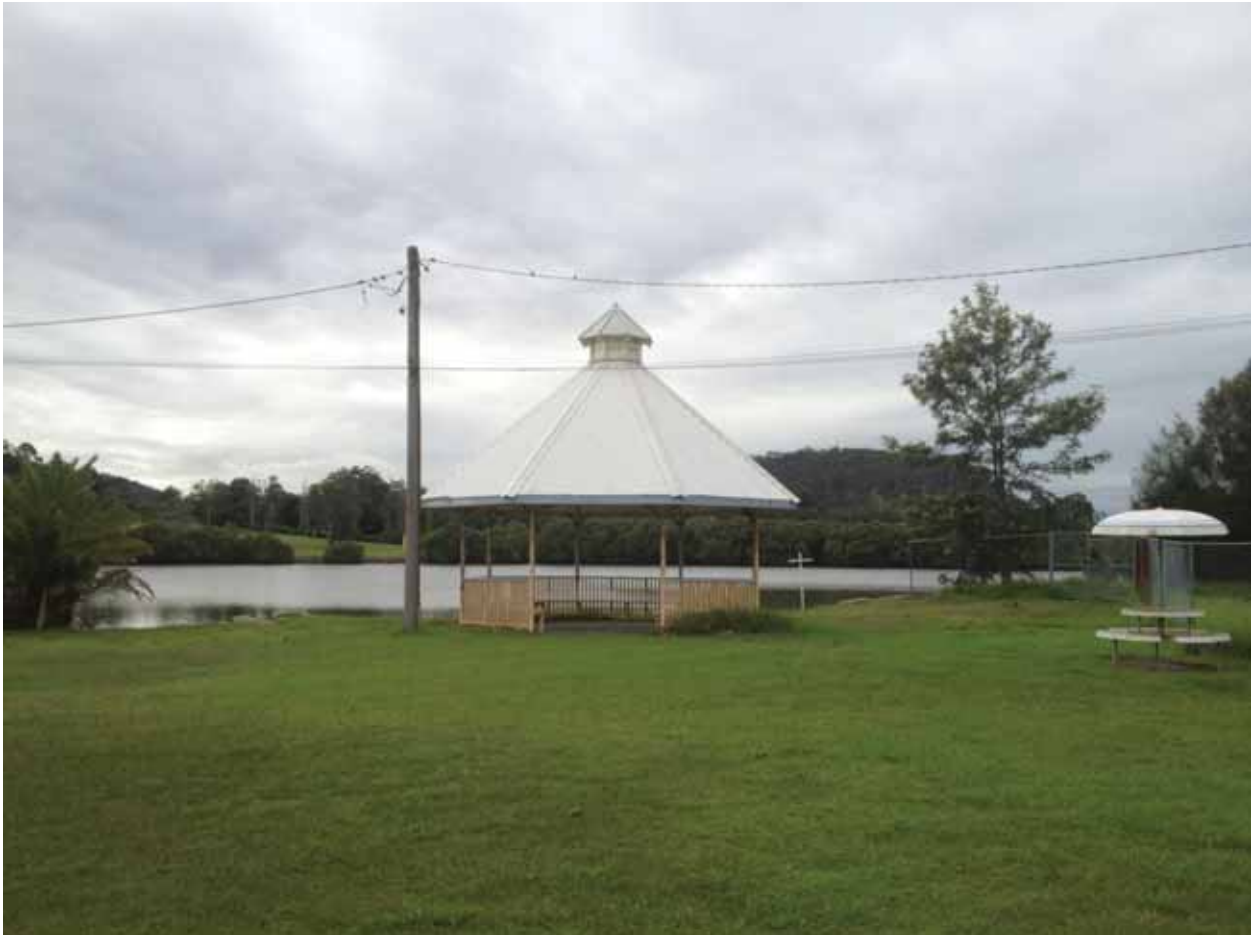
FIGURE 18 – EXISTING ROTUNDA (ITEM 21)
