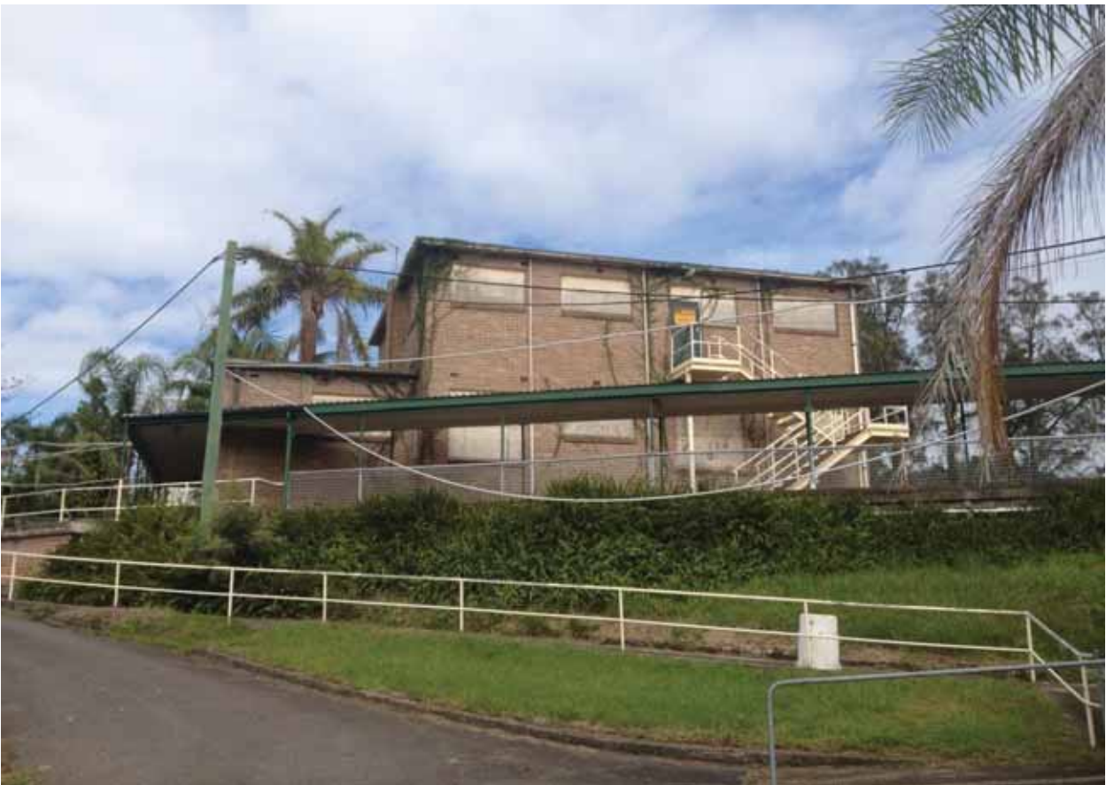
FIGURE 6 – VIEW WEST SHOWING EASTERN ELEVATION OF THE PINES BUILDING (ITEM 8)
