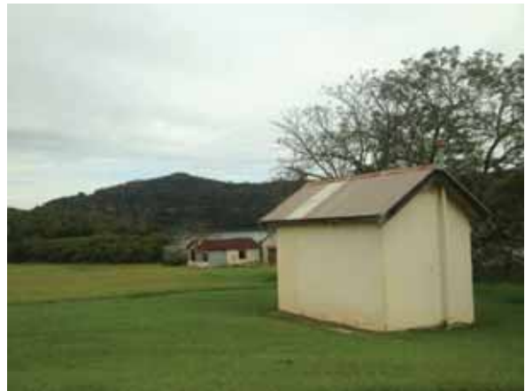
PICTURE 26 – SHED (ITEM 40)
