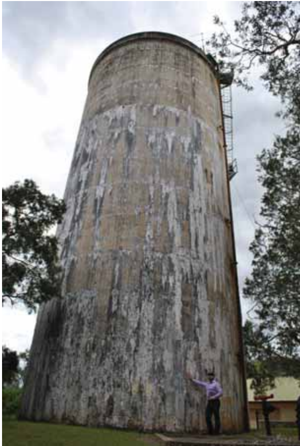
PICTURE 15 – WATER TOWER (ITEM 2)
