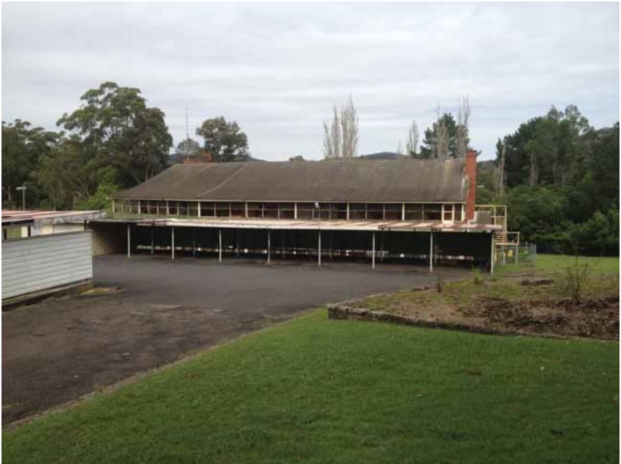
FIGURE 32 – FORMER STAFF QUARTERS BLOCK AND CAR PARK IN FOREGROUND (ITEM 36)
