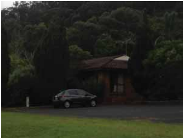
PICTURE 27 – VIEW NORTH SHOWING PRINCIPAL ELEVATION
