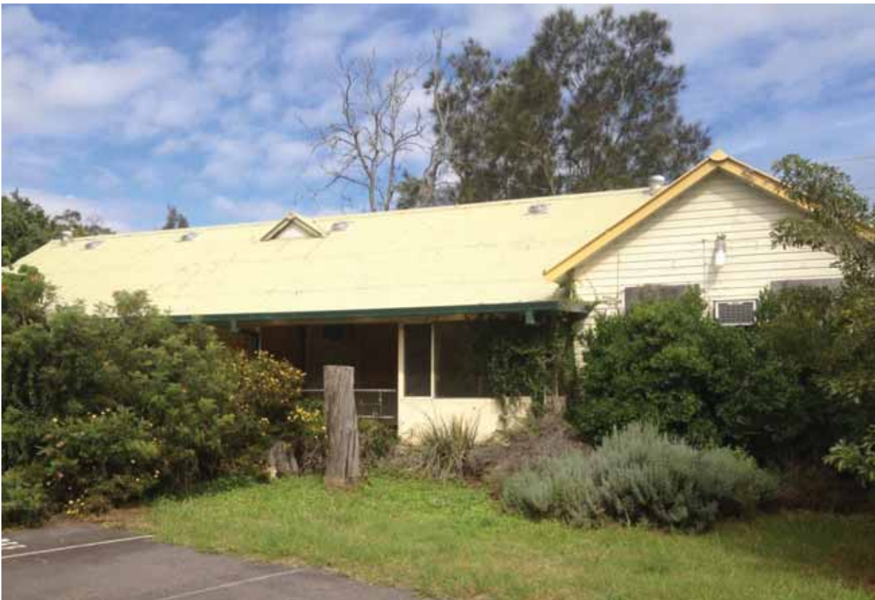
FIGURE 14 – VIEW WEST SHOWING EASTERN (PRINCIPAL) ELEVATION OF BINDAREE (ITEM 1)
