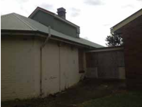
PICTURE 3 – KITCHEN LINK TO STORE ROOM
