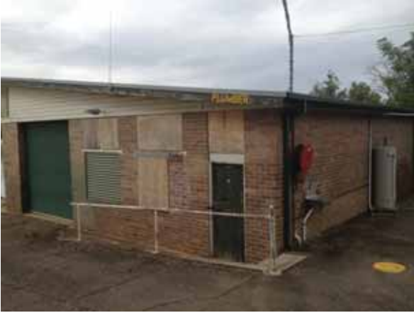
PICTURE 11 – PLUMBER'S SHED NORTHERN ELEVATION (ITEM 17)
