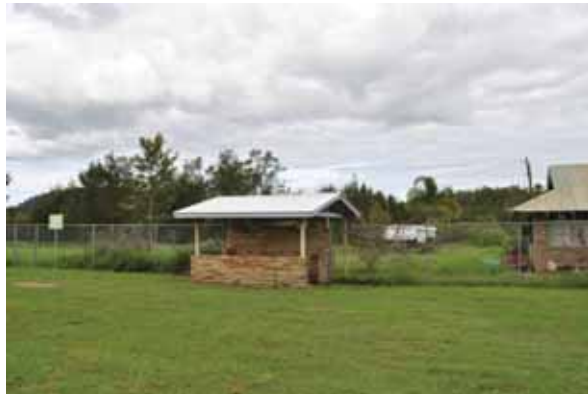
PICTURE 14 – SHELTER (ITEM 53)
