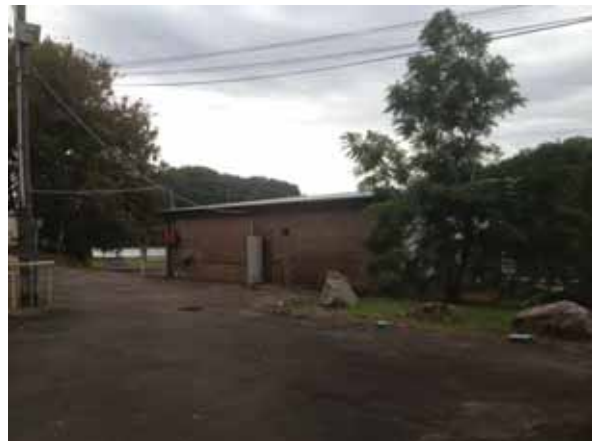
PICTURE 10 – PLUMBER'S SHED (ITEM 17)
