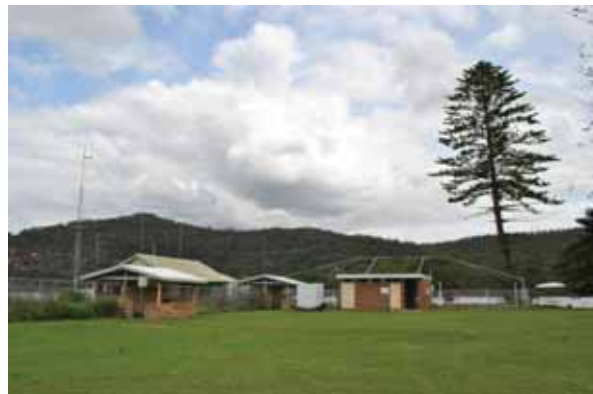
PICTURE 18 – LANDSCAPING INCLUDING SA SHED AND WASHROOM AMENITIES
