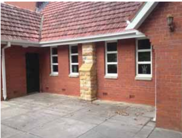
PICTURE 31 – EASTERN ELEVATION
