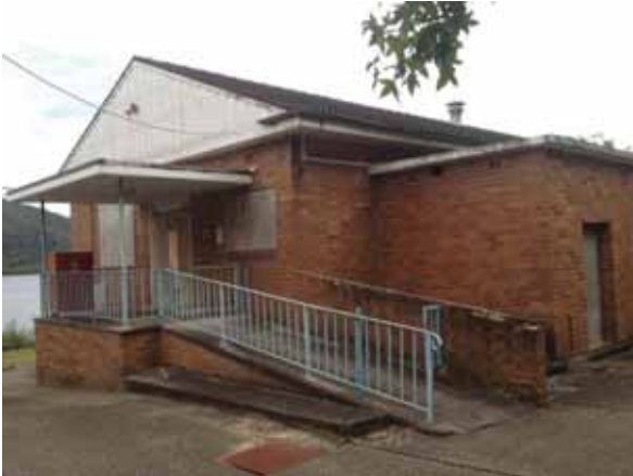
PICTURE 19 – SANBROOK BUILDING (ITEM 23)
