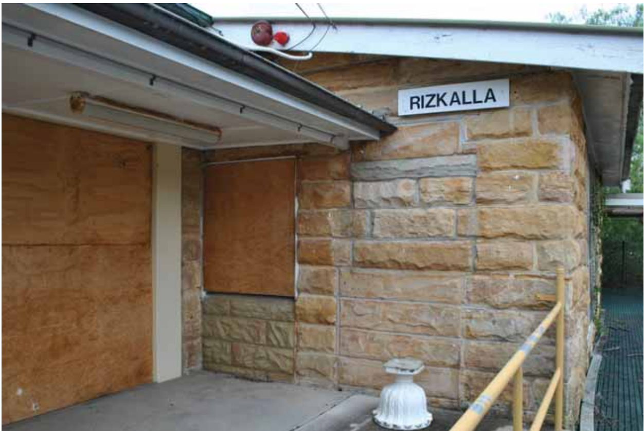
FIGURE 12 – RIZKALLA BUILDING (ITEM 5)
