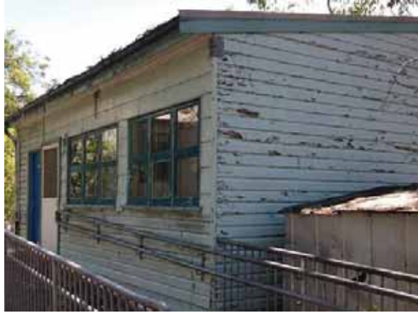
PICTURE 36 – CONDITION OF BUILDINGS
