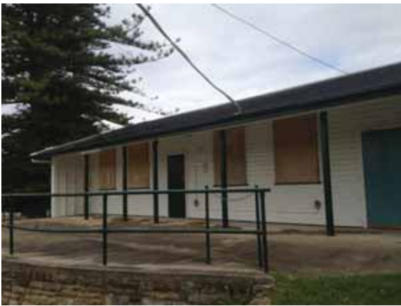
PICTURE 7 – EASTERN ELEVATION
