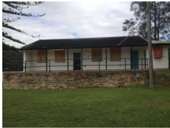
PICTURE 8 – EASTERN ELEVATION SHOWING SANDSTONE VERANDAH PLATFORM
