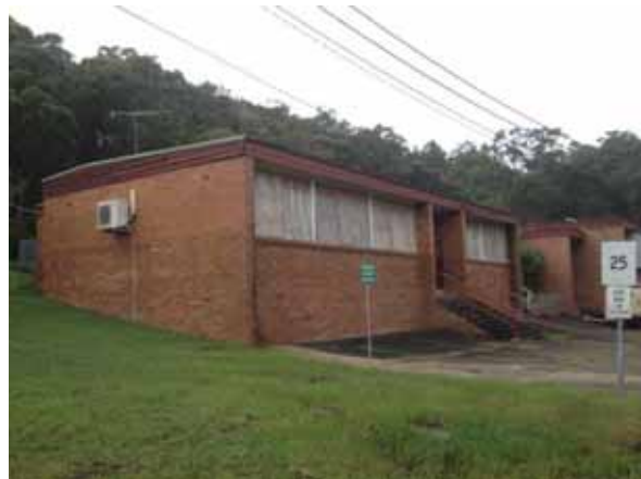
PICTURE 22 – CARPENTER'S BUILDING (ITEM 26)
