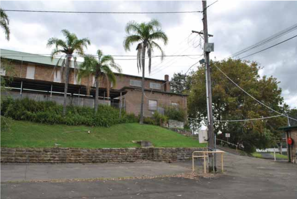
FIGURE 3 – SOUTH EASTERN ELEVATION OF SEA BREEZE (ITEM 13)
