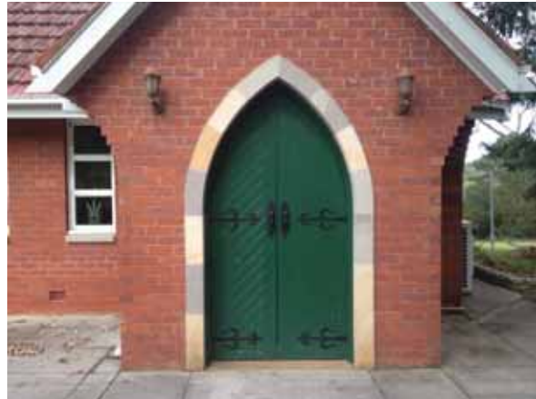
PICTURE 30 – EASTERN ENTRANCE
