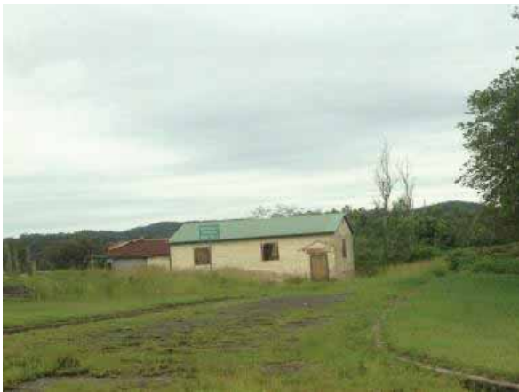
PICTURE 25 – VIEW SOUTH SHOWING DAIRY/SECONDARY STORES
